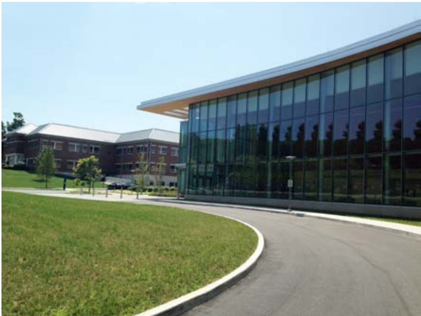
Fig. 2. Eastern's new Administration and Fine Arts buildings.
